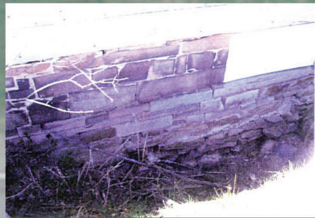
(b) VIEW OF FOUNDATION, CUT STONE AND MORTAR FOUNDATION
